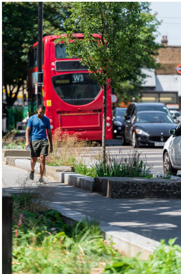
Photo: Retrofit bioretention raingardens alongside a busy high street with street tree planting.
