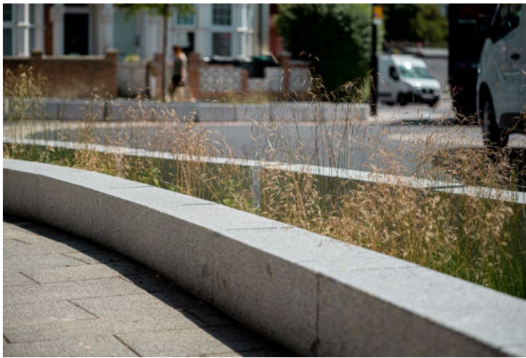
Image: Bioretention raingardens positioned between street/road and pedestrian pathway, constructed with robust, slotted roadside kerb inlets.
