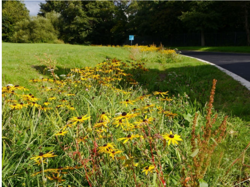
Image: A retrofit SuDS scheme featuring several bioretention raingardens specifically designed to collect and slow the ‘first flush’ of polluted runoff from the adjacent highway before the water is conveyed into secondary raingardens.
